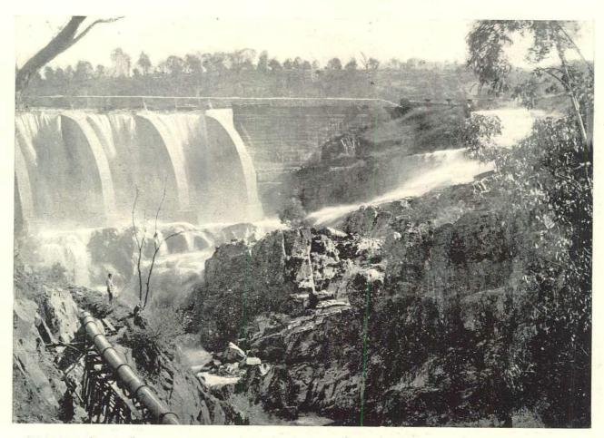
CARCOAR-GARLAND.-" JUNCTION DAM," BELUBULA RIVER, SHOWING BY-WASH AND PIPE-CONVEYING POWER TO THE 50-HEAD BATTERY AND PLANT OF THE LYNDHURST GOLD-MINING CO.
