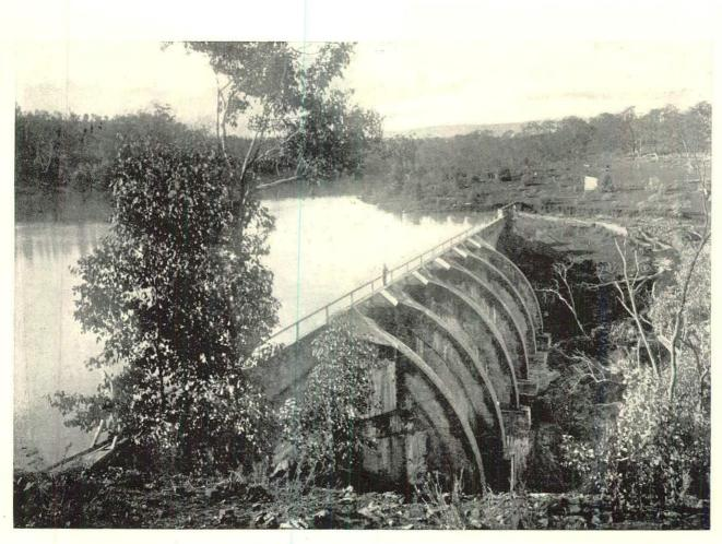
CARCOAR-GARLAND .- "JUNCTION DAM." BELUBULA RIVER. SHOWING THE DOUBLE ARCH PRINCIPLE OF CONSTRUCTION.
