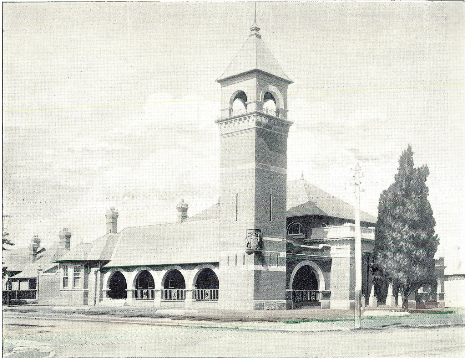
COURT HOUSE AND POLICE BUILDINGS, PARRAMATTA.
