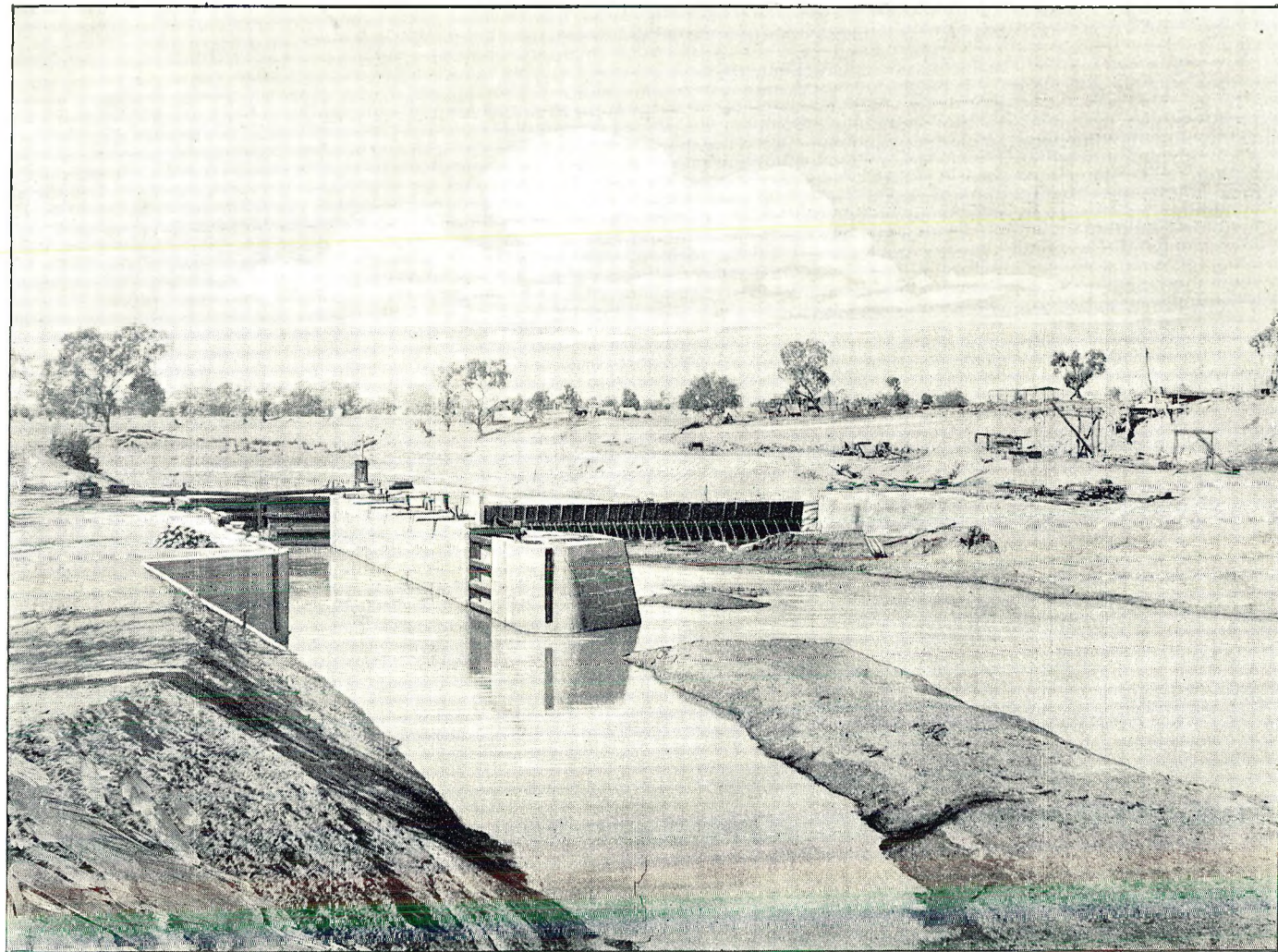
LOCK AND WEIR ON RIVER DARLING NEAR BOURKE, NEARING COMPLETION.
