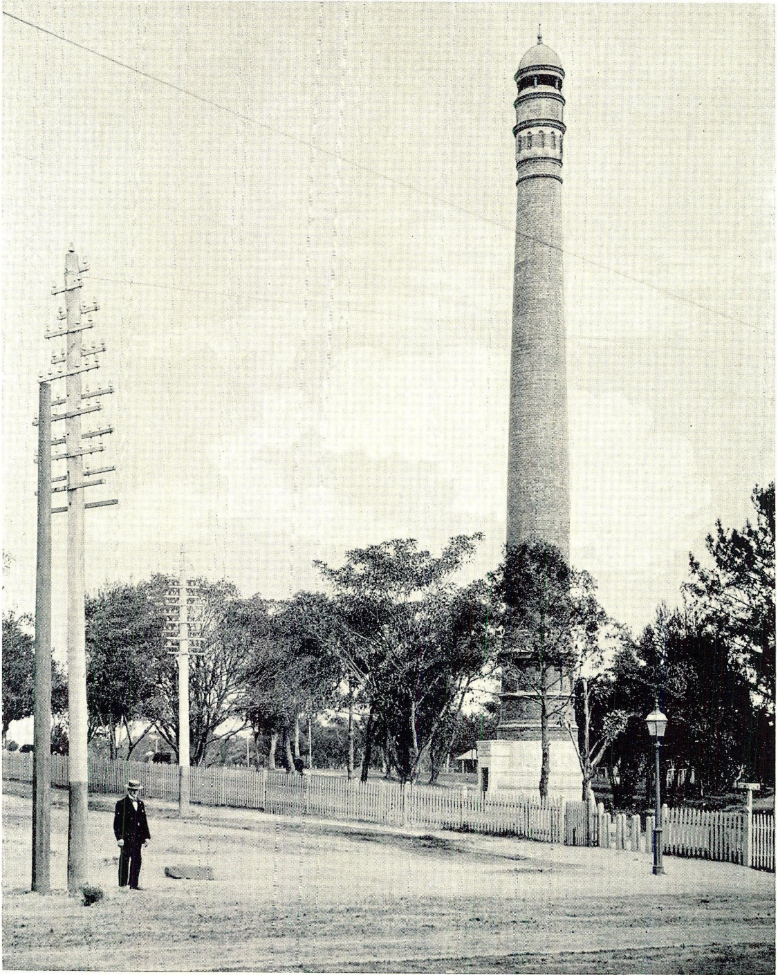
VENTILATING SHAFT, NORTH SYDNEY SEWERAGE, ST. LEONARD'S PARK.
